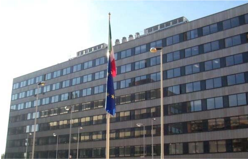
View of the ANPA's building
