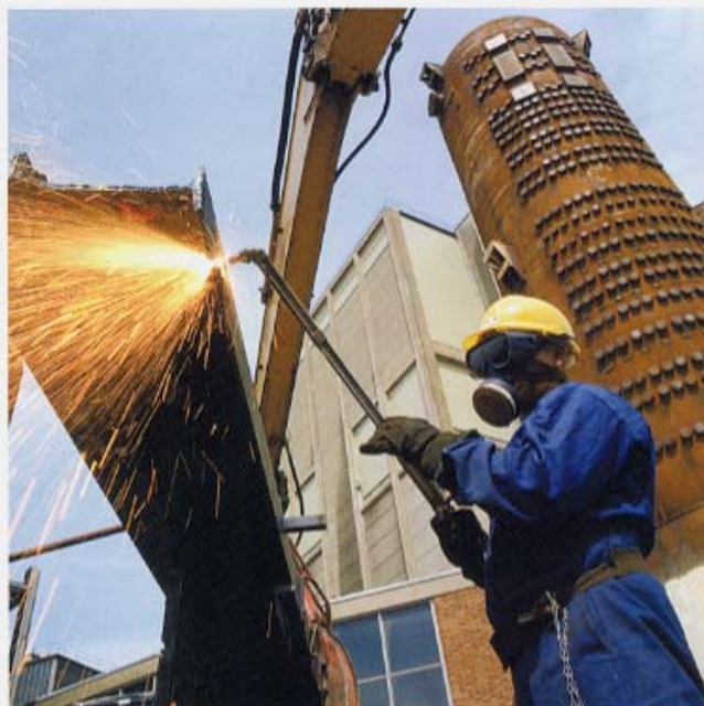
▲ Decommissioning activities at Berkeley nuclear power station.
