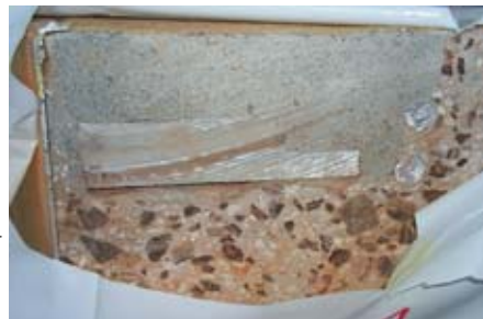
Cut through concrete and rebars
